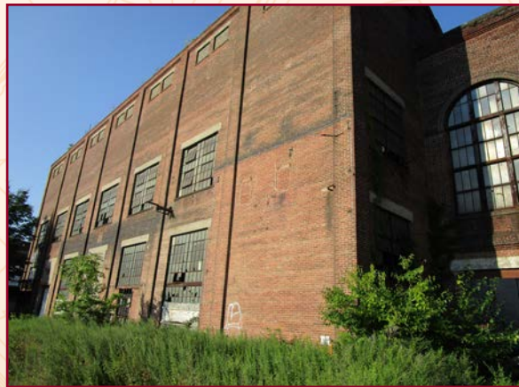
Elmer Street Boiler and Engine Room (Exterior)
